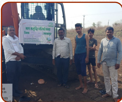
Strengthening community water structures for long-term impact.
